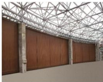
厦门海流飞机库大门 Hanger door in Xiamen Seaside
