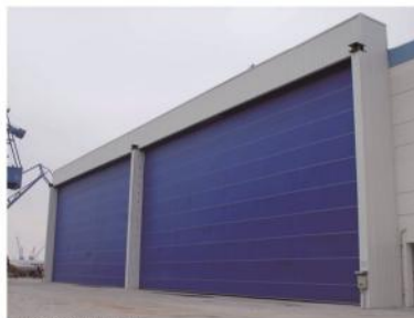
韩国24m×10m软帘上叠门 Korea 24m×10m soft curtain upper folding door of opening
