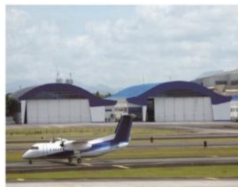
菲律宾机场大门 Hanger door in Xiamen Seaside/Philippine Airport door
