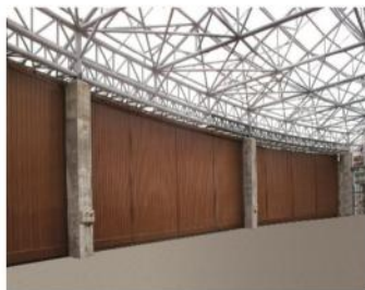
厦门海滨飞机库大门 Hanger door in Xiamen Seaside
